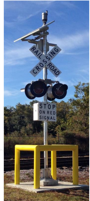
Industrial Area Crossing Signal with 4 Lights
