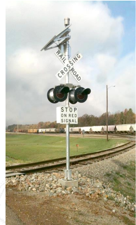
Industrial Area Crossing Signal with 4 Lights
